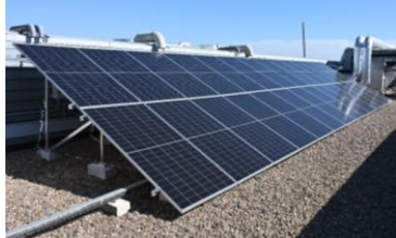
Photovoltaic generation (4x15kWp)
