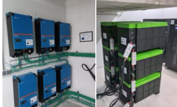
Batteries storage (80.64kWh)
